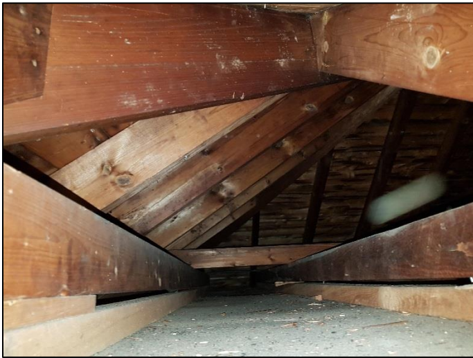
Photo 6: Existing Roof Construction
