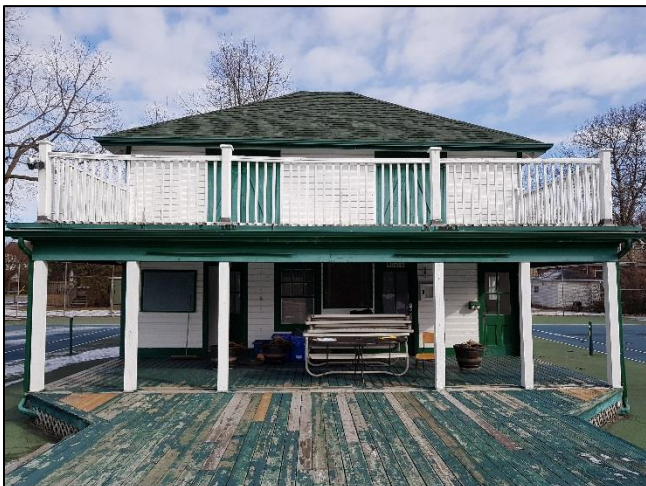
Photo 1: Original Main Building
