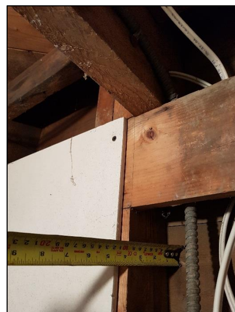
Photo 5: Typical Joist to Stud Wall Connection
