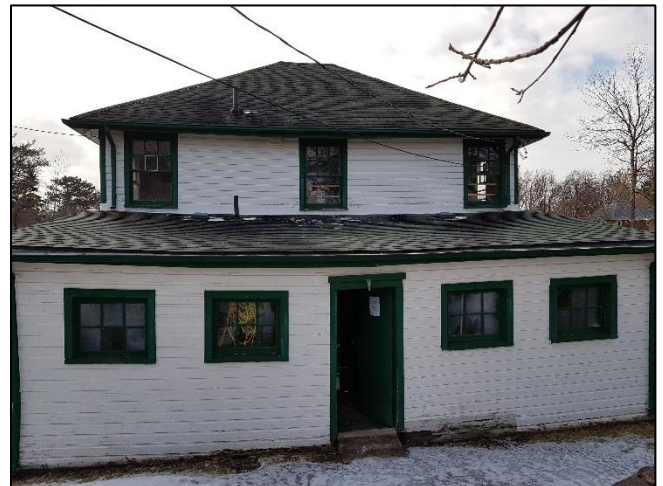
Photo 2: Rear Storage Shed Addition
